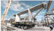
Coupled laterally here, two PowerHoss modules are transporting 175 t bridge segments to the girder launcher.
